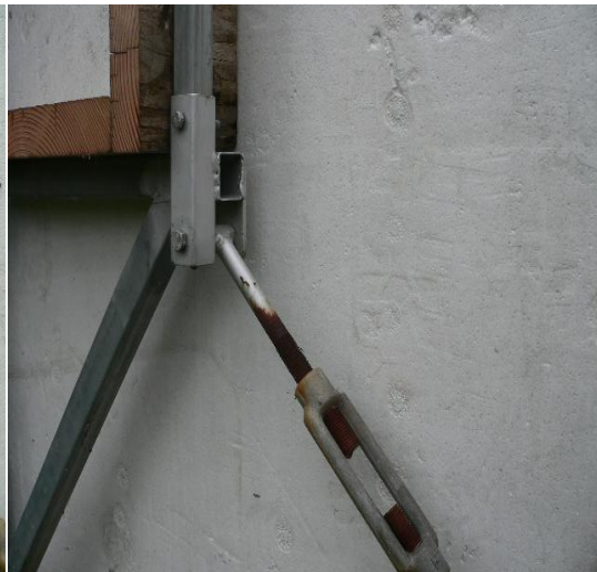
Adjust turnbuckle to plumb wall.
