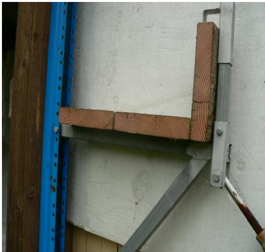
Positioning of planks and kickboard.
