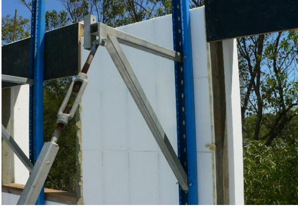
When fixing Strong Back to floor with 6.5mm blue concrete screws.
