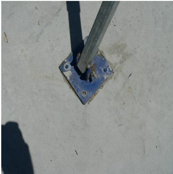
Fixing brace to concrete floor.
