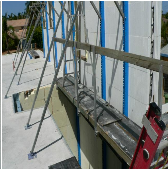
Putting braces from bottom to top through stairwell.
